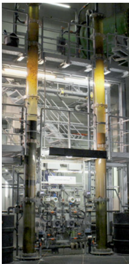
Fig. 5.3: Technical barriers in drinking water treatment: pilot rapid filter at the OWA in Berlin-Tegel, joint research project ASKURIS
