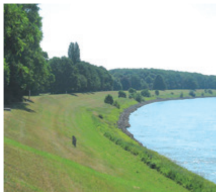
Fig. 5.1: Bank filtration on the Rhine (Düsseldorf) – natural barrier for safe drinking water (© TZW, Karlsruhe)
