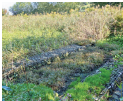
Fig. 3.3: Microbiological assessment concepts facilitate evidencing the effectiveness of constructed wetlands, for example (© M. Scheurer, TZW, Karlsruhe)
