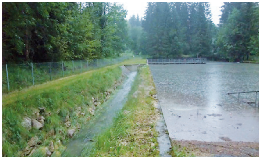
Fig. 5.5: Overflow of the storm water retention basin (combined sewer system) after heavy rainfall (© C. Stange, TZW: DVGW-Water Technology Center, Karlsruhe)
