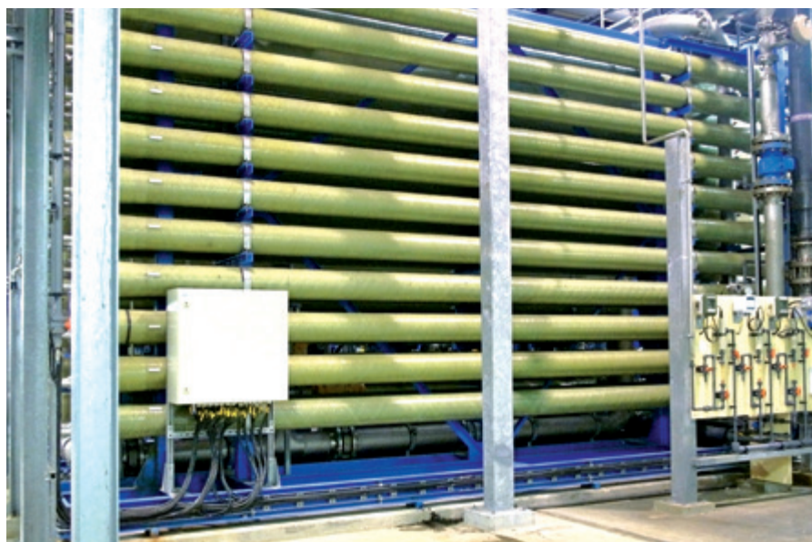
Fig. 4.3: Ultrafiltration membranes for the treatment of surface water (© DEHEMA, Frankfurt am Main)
