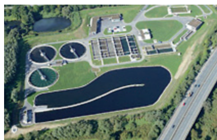
Fig. 2.2: Municipal wastewater treatment plant (© Ruhrverband, Essen)
